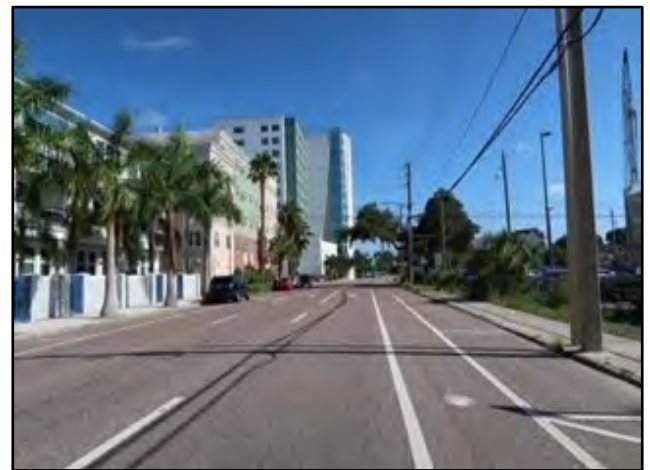
VIEW NORTH ALONG 8 TH STREET
