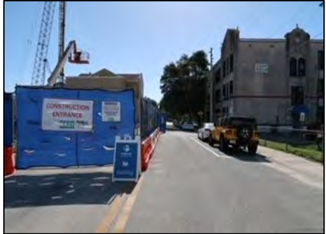
VIEW EAST ALONG 3 RD AVENUE
